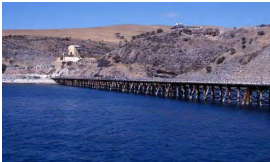
Rapid bay jetty is well over 400 meters long
